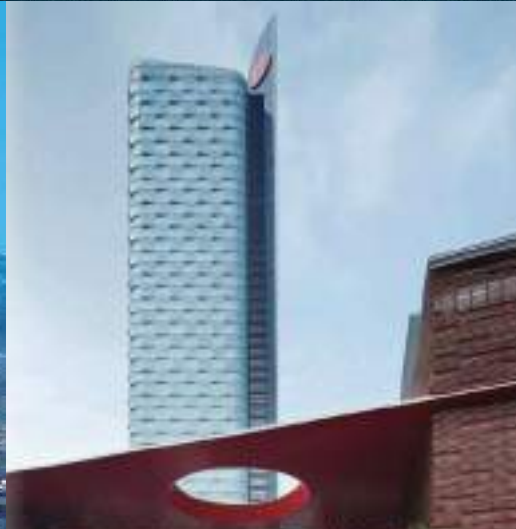
Citic Plaza (Office Building) Shanghai, China 2011
